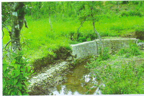
Fig. 2. Stone masonry and gabion retaining wall (Mawpun)
