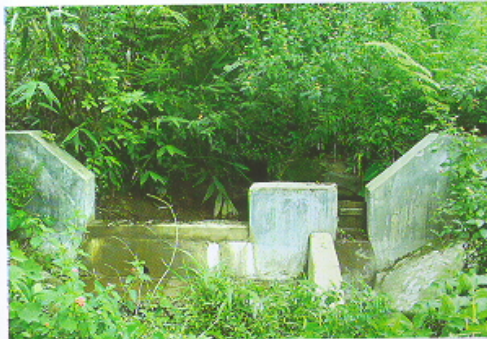
Fig. 3. Rectangular weir cum diversion wall (Mawpun)
