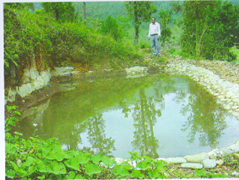
Fig. 5. Plastic lined pond at hilltop (Mawpun)
