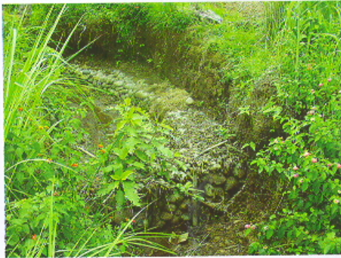
Fig. 1. Check dam -Gabion (Mawpun)
