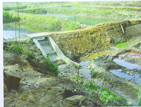
Fig. 6. Earth dam and masonry chute spillway (Mawpun)
