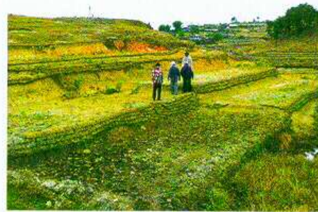
Fig. 14. Newly constructed terraces at the Watershed site, Mawlangkhar
