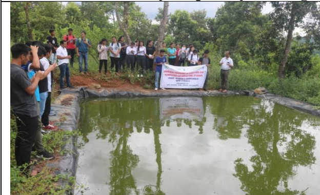
Water harvesting structure jalkund for multipurpose use
