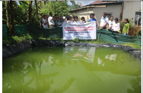
Water harvesting structure jalkund for multipurpose use
